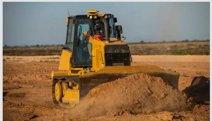
SITE PREPARATION - COARSE GRADING
